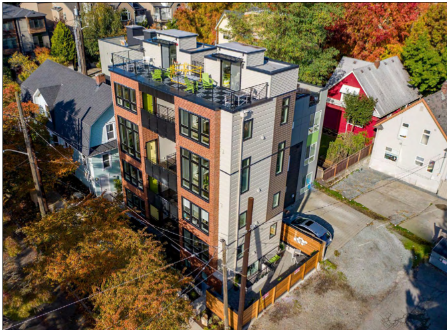
A multifamily building in Seattle with a single staircase, which allows for construction on smaller parcels and more diverse unit configurations serving a broader range of needs. Photo source: Sean Jursnick/X.
